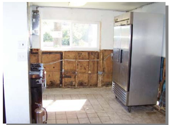
Looking towards the front of the house in the Kitchen.
